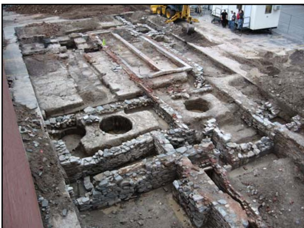
1: Overall view of the site area showing foundation walls and backyard features.
