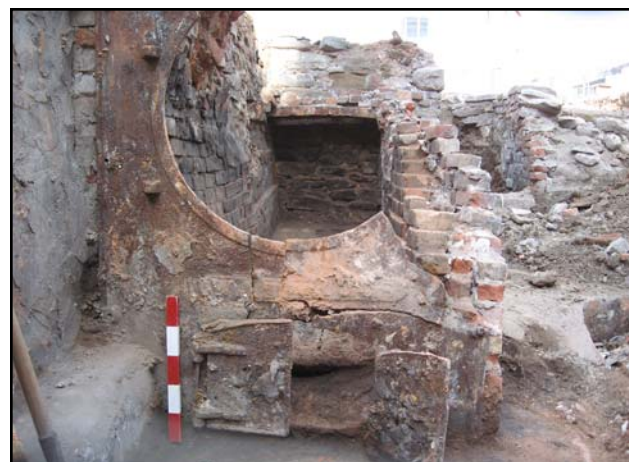
2: The basement of House 4 modified to hold a large coal-burning furnace.
