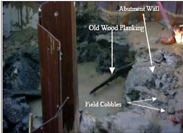
**Figure 4: Old Wood Planking from South Bank Wing Wall**
