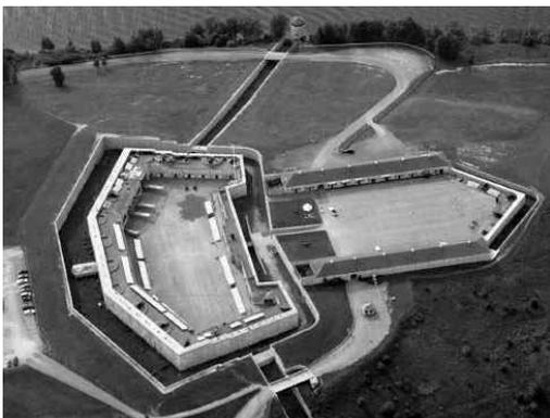
**Figure 1.** Aerial view of Fort Henry seen from the west. The enclosed redoubt is to the north (left) and the advanced battery to the south (right). Photo by B. Morin. Parks Canada, Ontario Service Centre [OSC], Cornwall. Photo no. 131H-457E.
